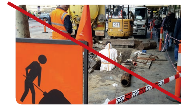
Easy rehabilitation without digging
